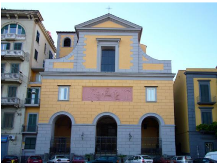
A recent picture of the façade of the church of San Giuseppe a Chiaia
